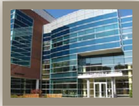
The newly renovated Klau Library at HUC
